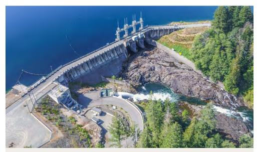
Site work has begun to prepare the area around the John Hart Dam in Campbell River for the upcoming John Hart Dam Seismic Upgrade Project. The Project includes seismic upgrades to strengthen the dam so it can withstand a severe earthquake. For more information on this project, as well as the Ladore and Strathcona projects, visit majorprojects.ca
